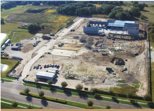
LifeLink Tissue Bank building progress. January 2009 Doria Photo Inc.
